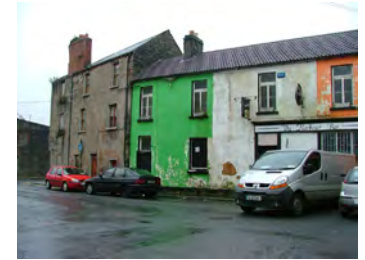
Derelict Buildings on Lower Quay Street
