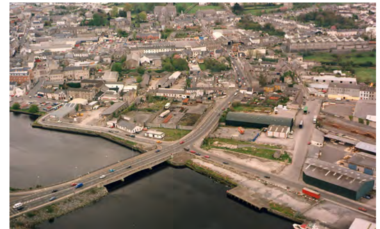
Aerial View (picture taken in September 2002)
