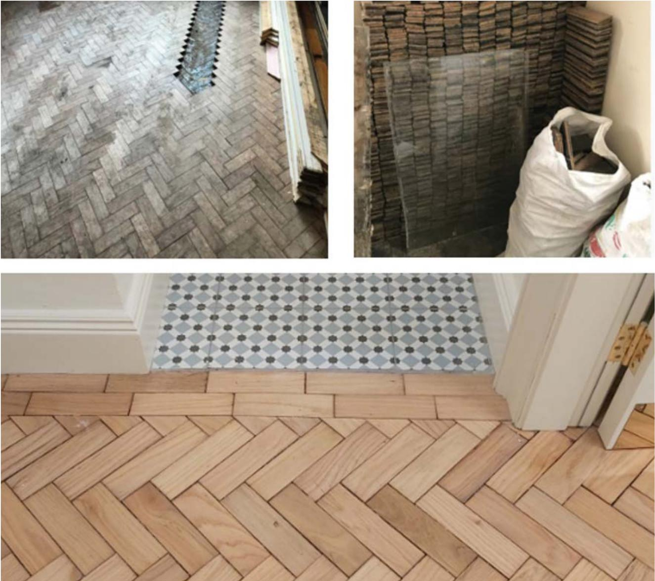
**Figure 4-2:** Reuse of flooring
